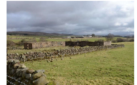
Figure 4.8: Rack Farmstead (looking northeast)
