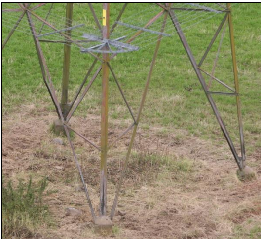
Figure 7 - U057 Bent Bracing Steelwork
