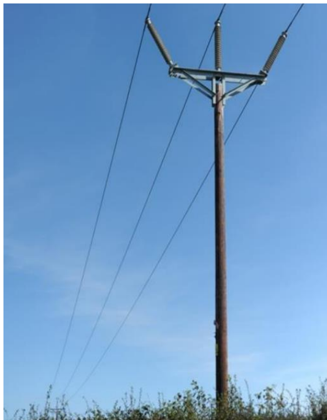
Figure 2. Typical Trident Wood Pole
