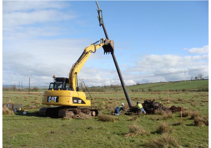
Photo 3.2: Erection of Wood Pole
