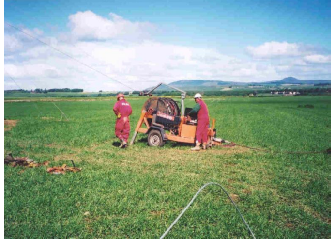
Photo 3.3: Conductor Stringing Winch
