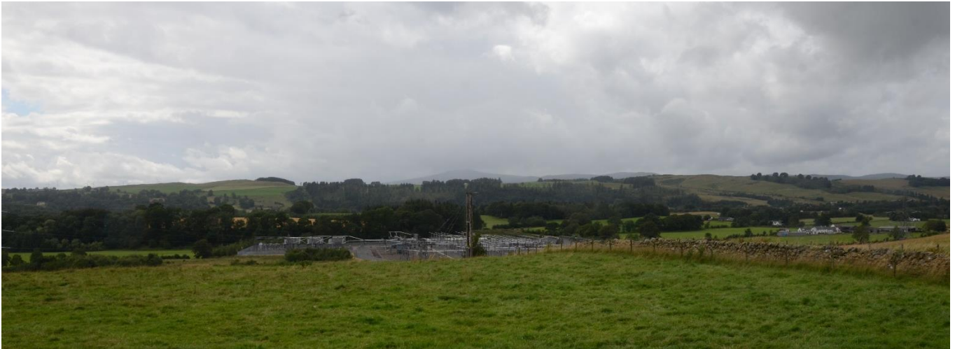
View west from road across towards Bearholm Substation and Milton (SM676) beyond.
