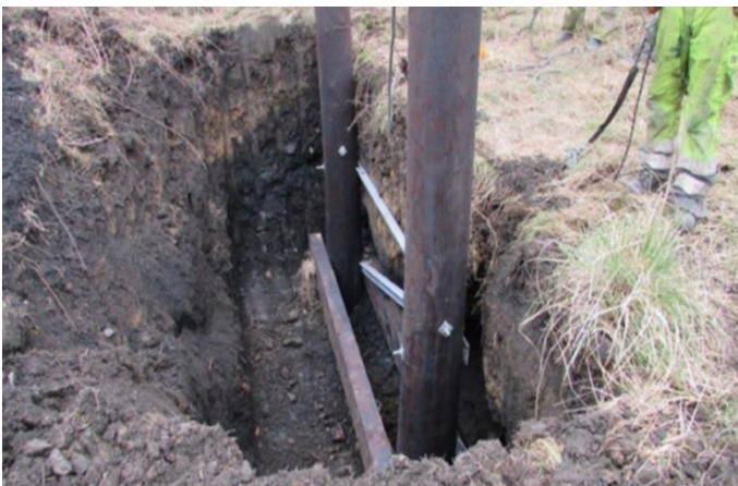
Photo 3.1: Typical Double Wood Pole Foundation Excavation
