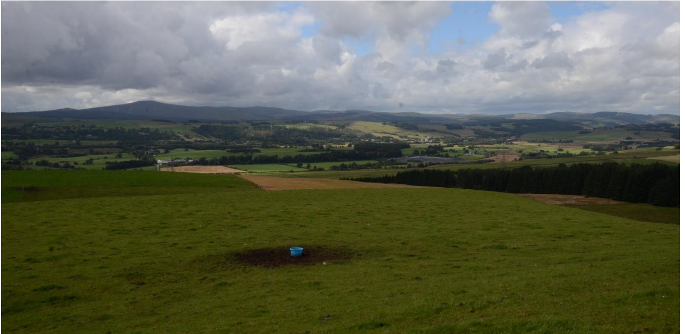
View westwards from the Dod, the Bearholm Substation in the middle distance on the right (north) of the image, and views of Hareshaw Rig beyond
