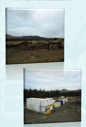
Work underway at the substation location includes the installation of a site compound with temporary offices. Work has also started to clear and level the area that will create the concrete platform. This platform will provide the base for the substation and house the mechanical and electrical infrastructure to be installed.
