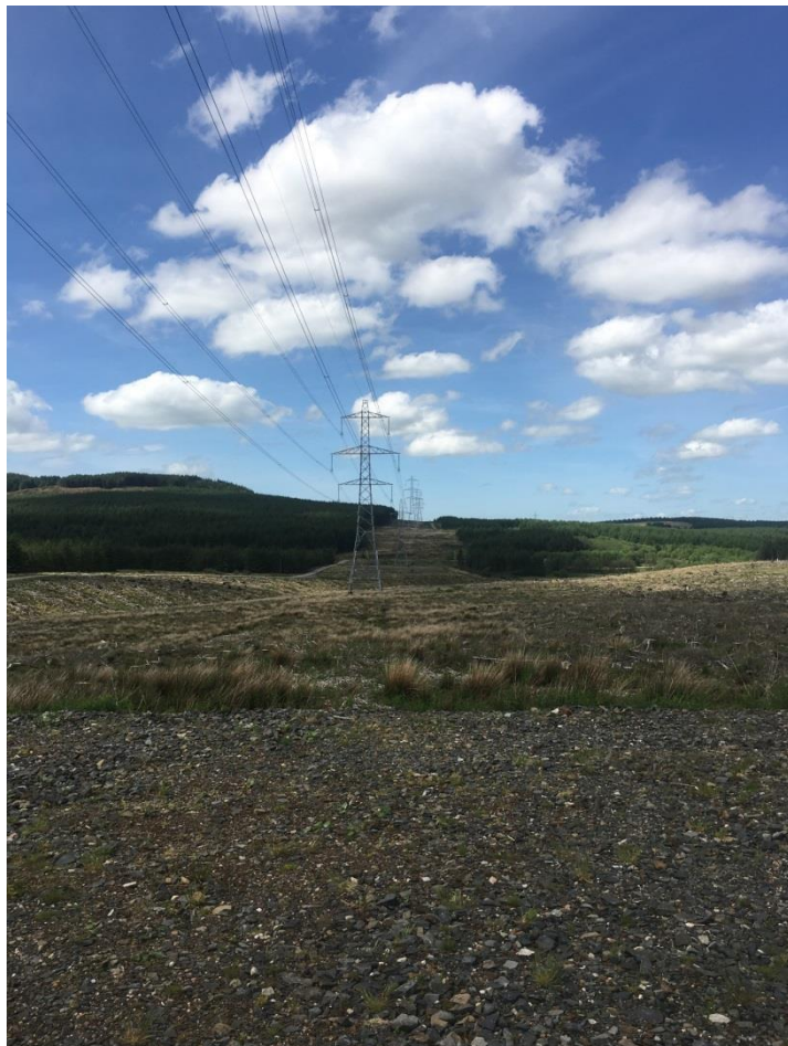
View of the recently installed 275kV WA Overhead Line between Coylton and New Cumnock substations
