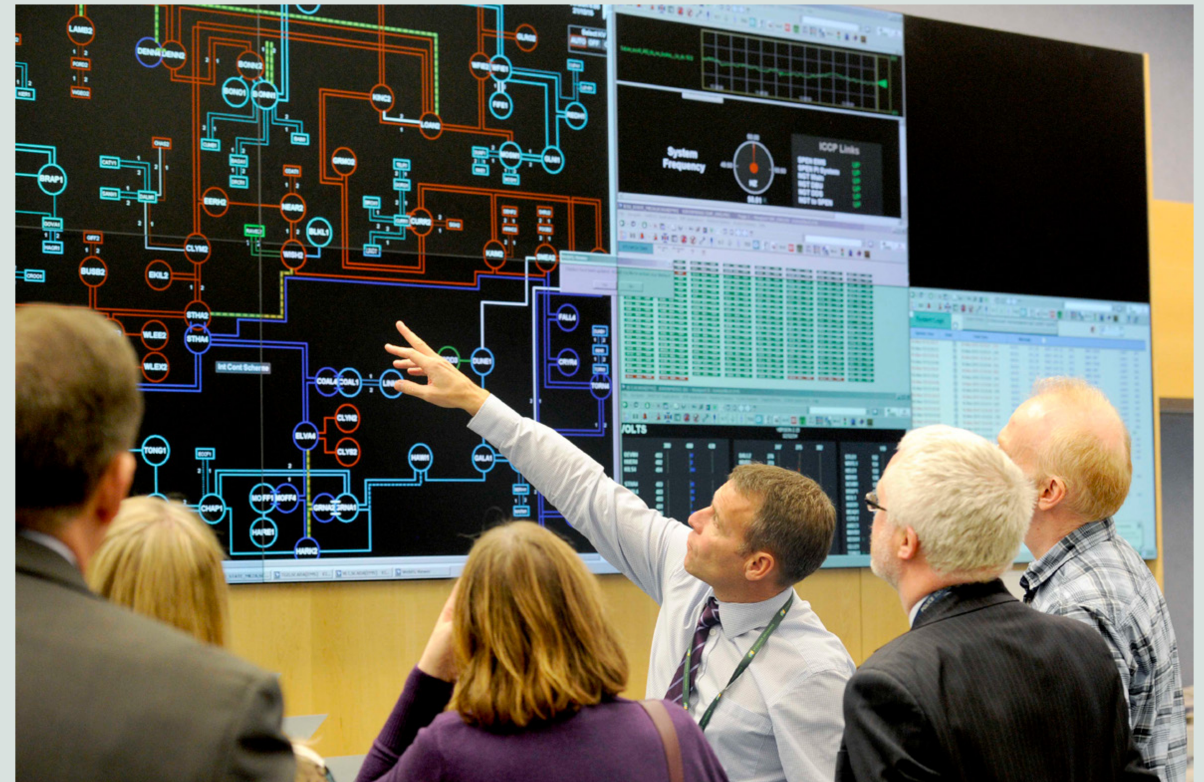
SP Energy Networks control centre in Glasgow
