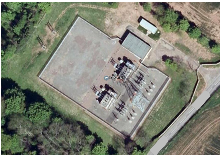
Dunbar Grid Supply Point
