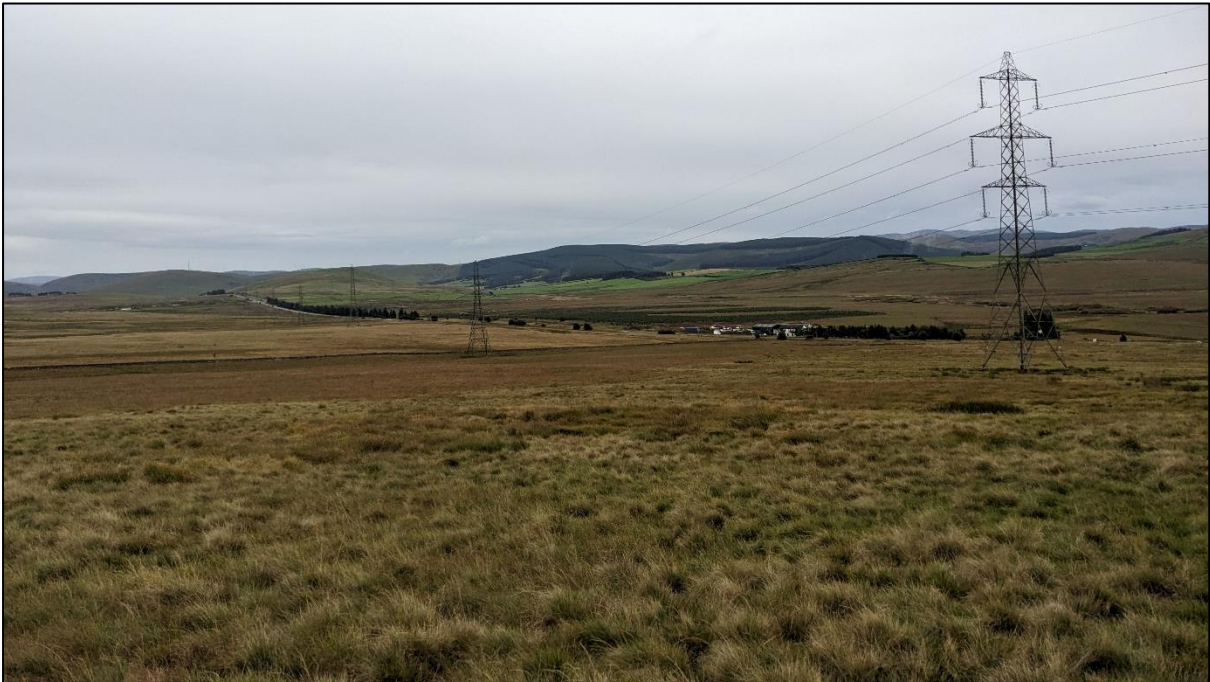
Photo 3-B: Site Condition (looking south-east from northern boundary)
