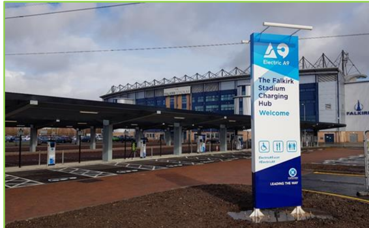
Figure 20 Electric A9 – Falkirk Stadium Charging Hub
