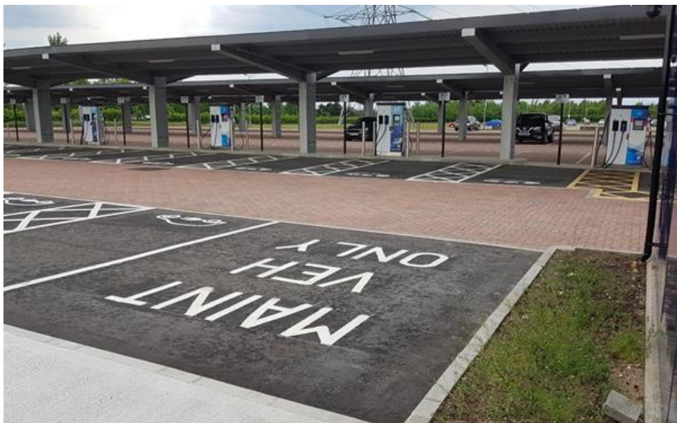
Figure 23 LV Engine Substation location at Falkirk
