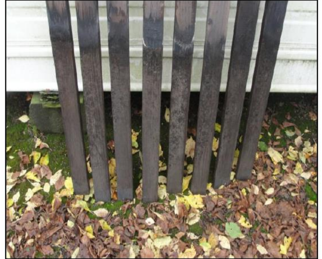
Creosote treated unsleeved stakes at 48 months: no overt indications of decay noted on these stakes.
