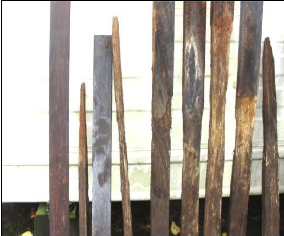
Untreated control stakes at 48 months: evidence of fungal decay and very significant timber loss. 50% failed completely at ground level during uplift.
