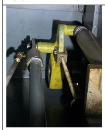
See the hole where the operating shaft should fully enter (flush to the end) / protrude through the yellow/red drive crank
