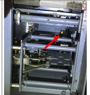
It is essential to focus in on the drive crank (typically yellow or red) to assess the units.
