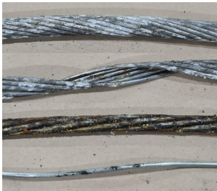
Figure 12 132kV Conductor Sample evidence on BE Route
