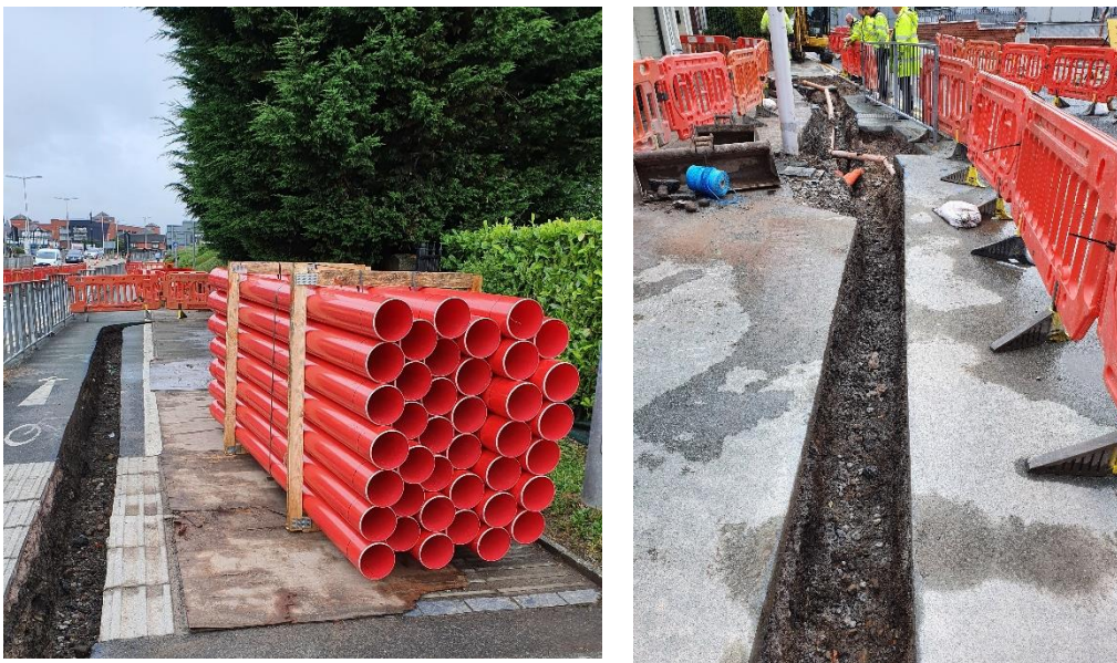
Figure 9 Small section cable upgrade between Crescent Road and Bingo Club substation
