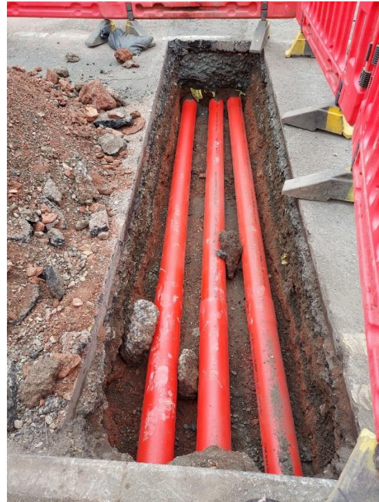
Figure 10 HV duct road crossing for Falkirk Stadium
