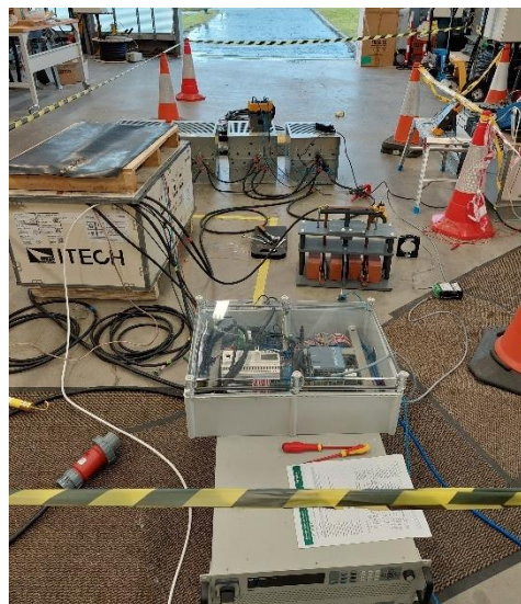
Figure 11 Short circuit withstand tests for earth leakage relays in PNDC
