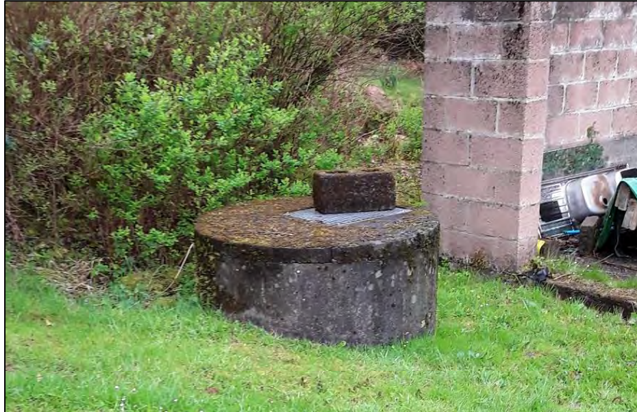
Photo 2: Covered manhole at Summerhill PWS location; potential well
