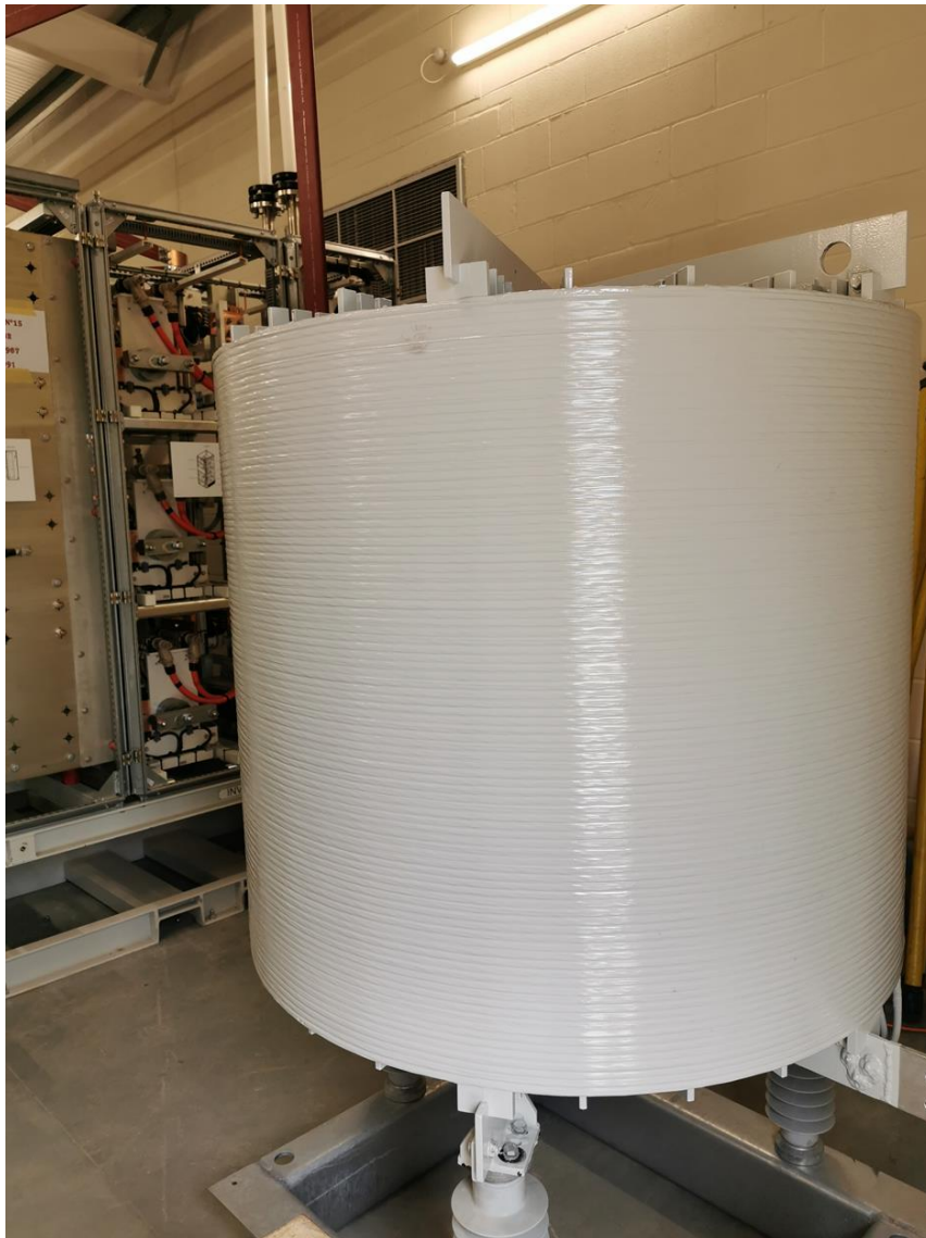
Figure 7. Mechanically installed DC reactor with DC solid bus connection completed.
