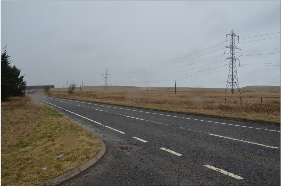
ZV Route (400kV England-Scotland Interconnector) from the B7080 near Red Moss
