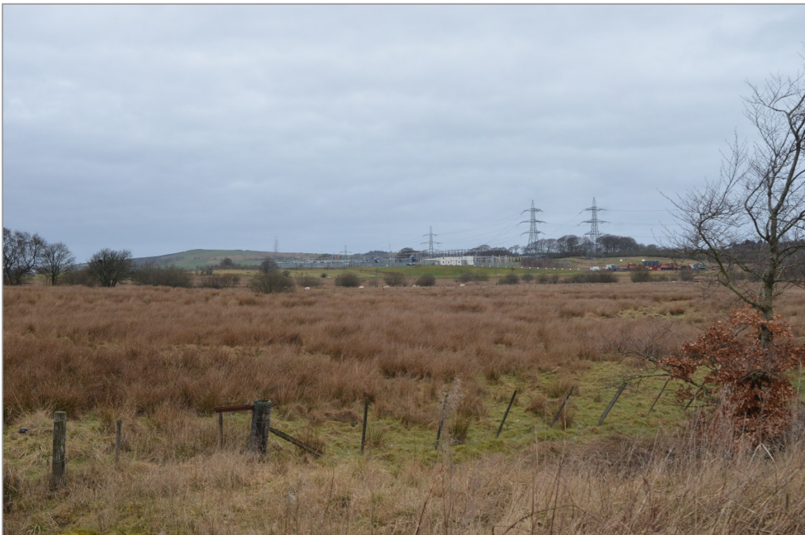
Coalburn Substation and ZV Route from the B7078
