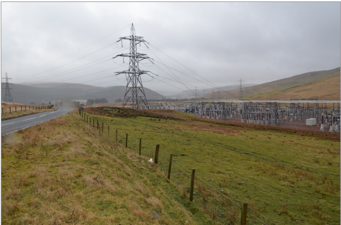
Elvanfoot Substation and ZV Route from the B7040
