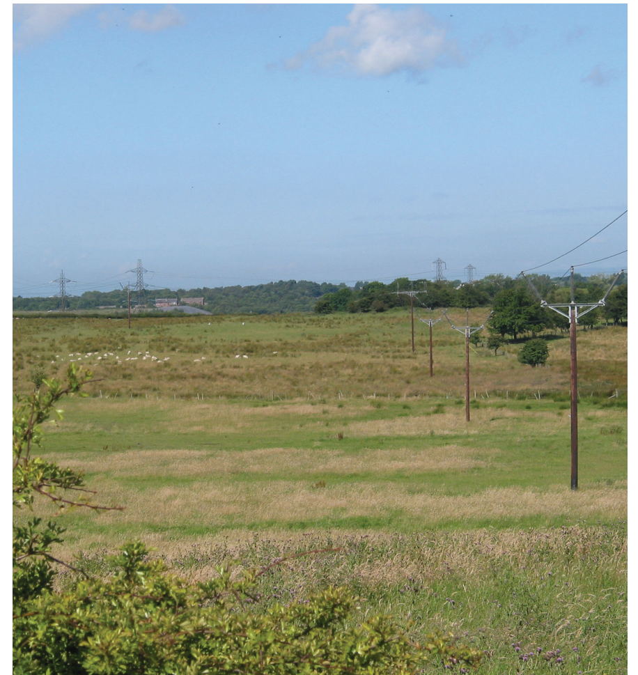
Trident single poles in lowland setting with lattice towers
