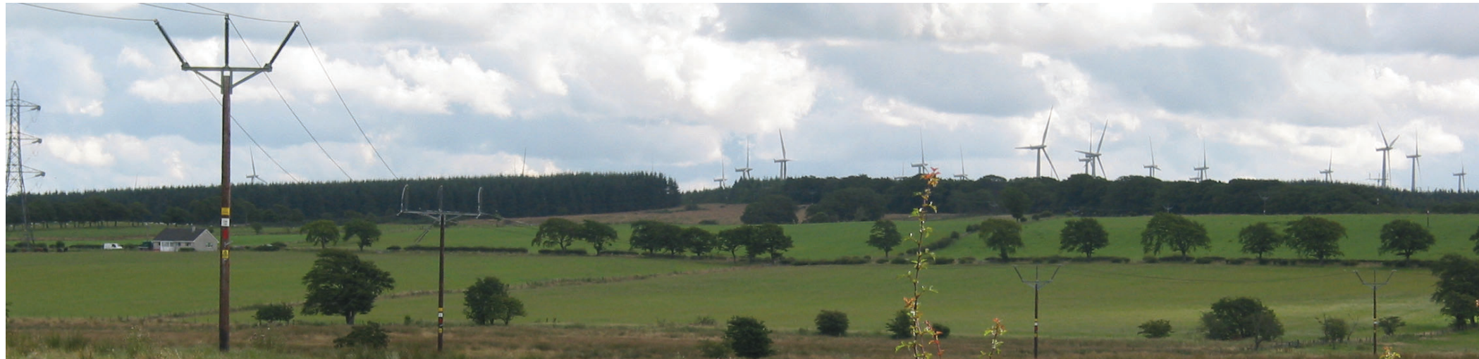
Trident single poles in lowland setting, with wind farm
