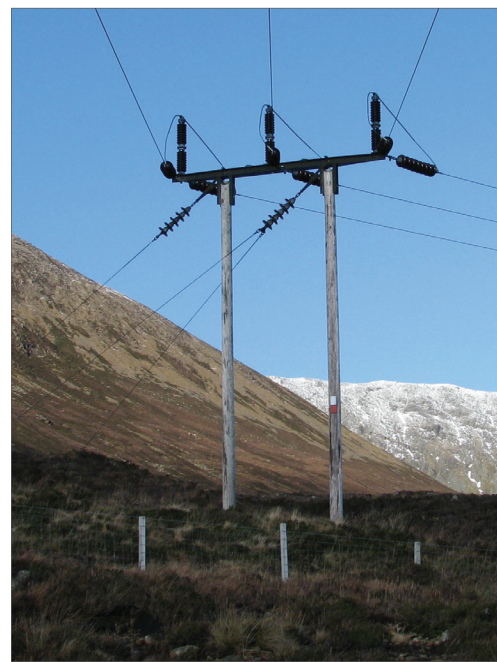
Trident 'H' pole turning pole
