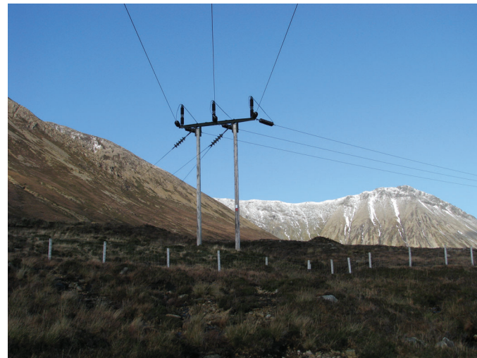
Trident 'H' turning pole in moorland setting
