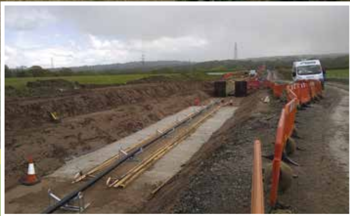
Cables will be installed underground
