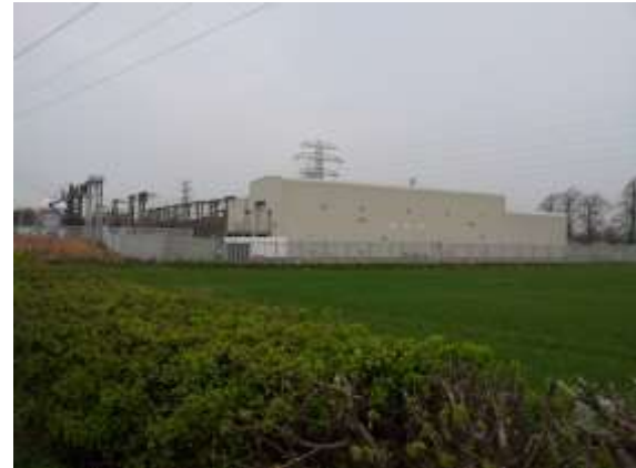
Figure 3.4: A typical 132kV GIS Building. It should be noted that the proposed substation at Kincardine would have a capacity of 275kV and would therefore be larger in size.
