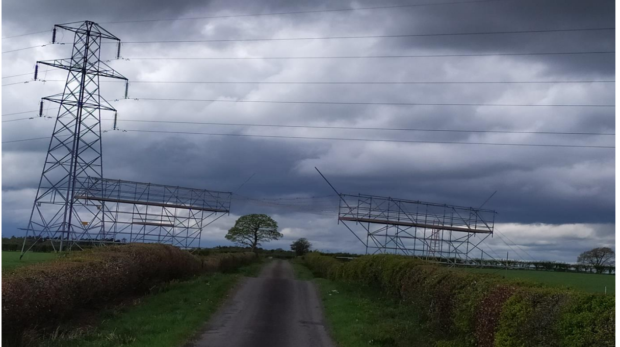
Illustration of a Scaffolding setup for Distribution/Transmission/Telecom crossing
