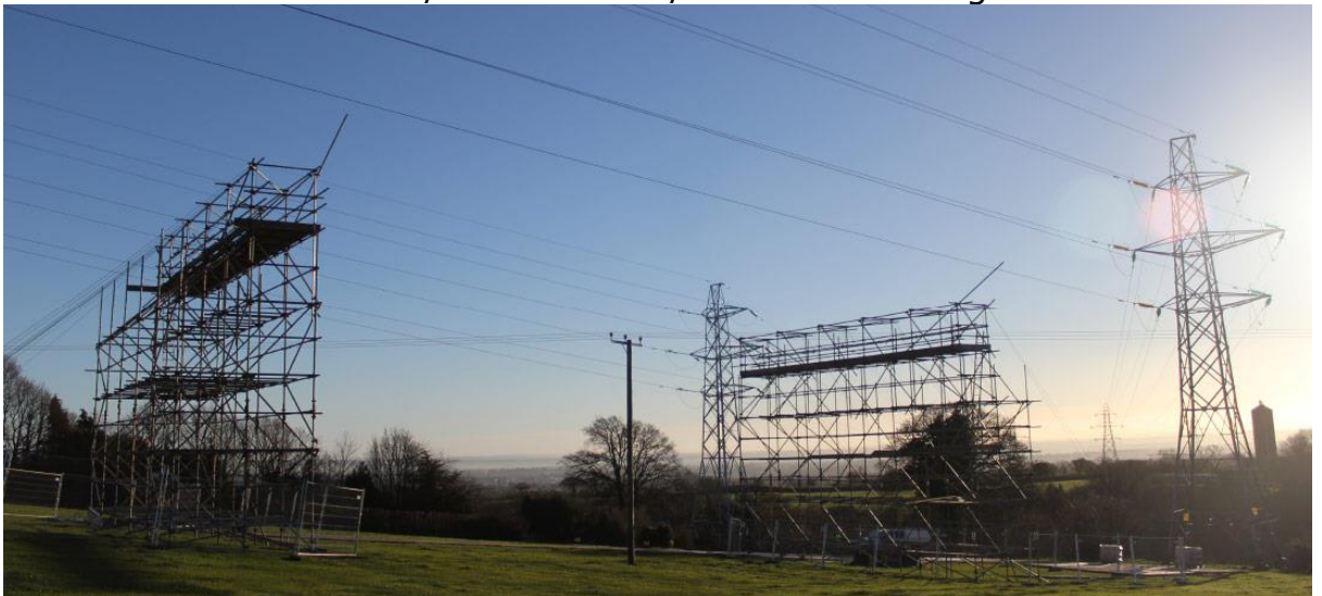
Illustration of a Scaffolding setup for Distribution/Transmission/Telecom crossing
