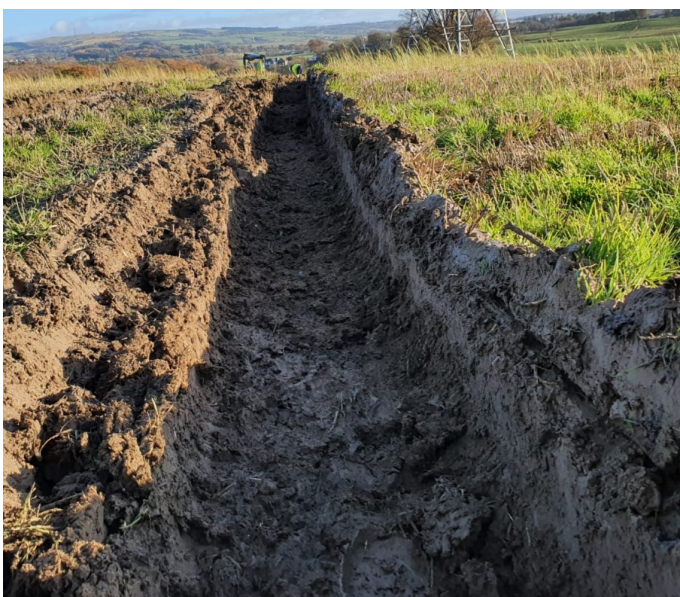
Significant ruts from machine access
