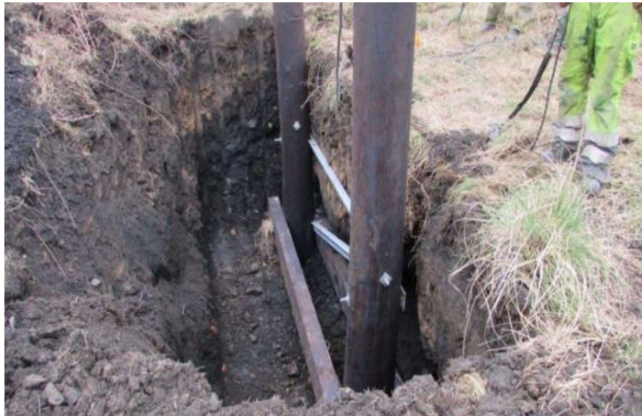
Figure 4.20: Typical wood pole foundation excavation
