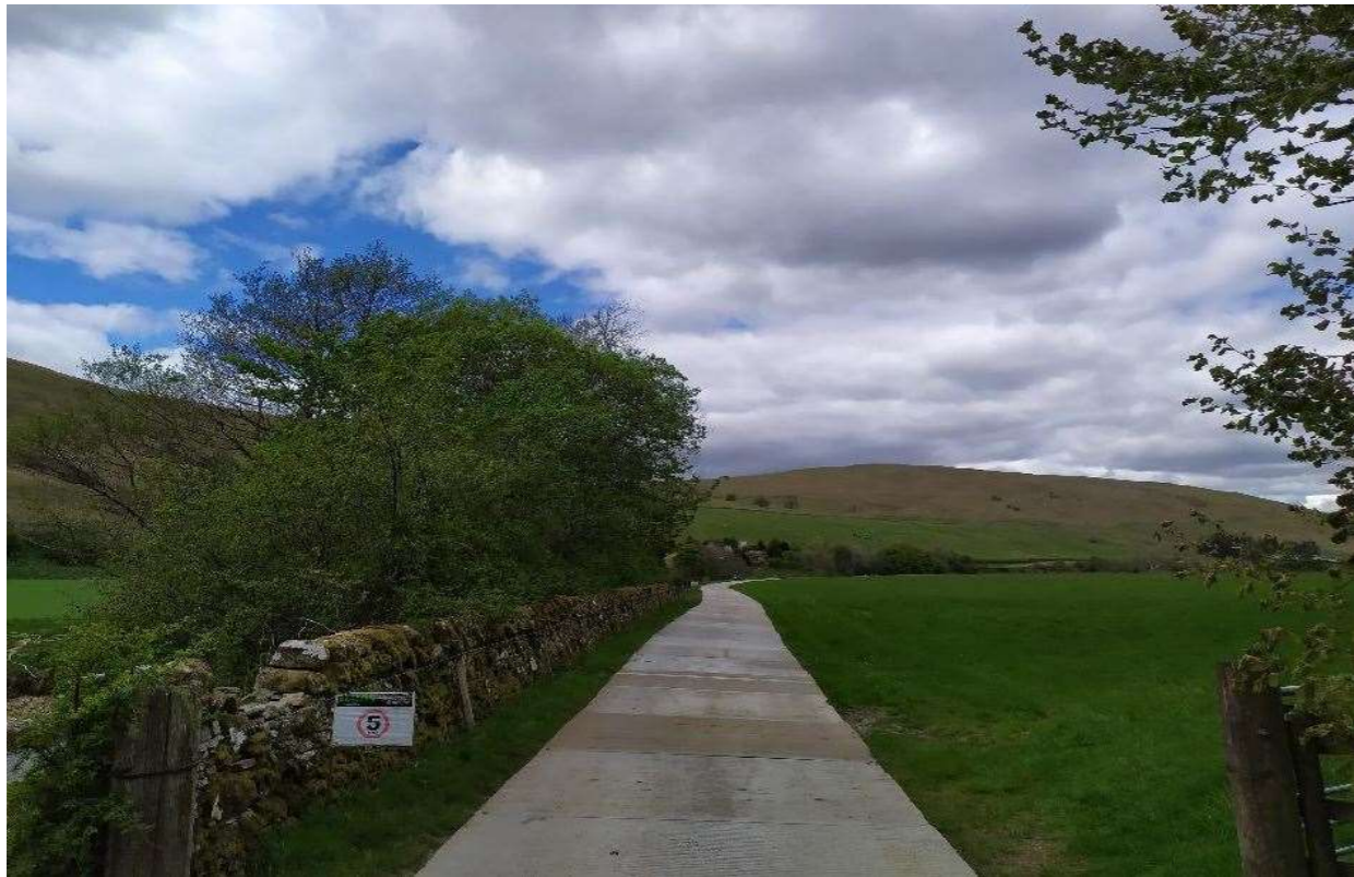
Figure 4.12: Typical trackway panel/Terrafirma installation
