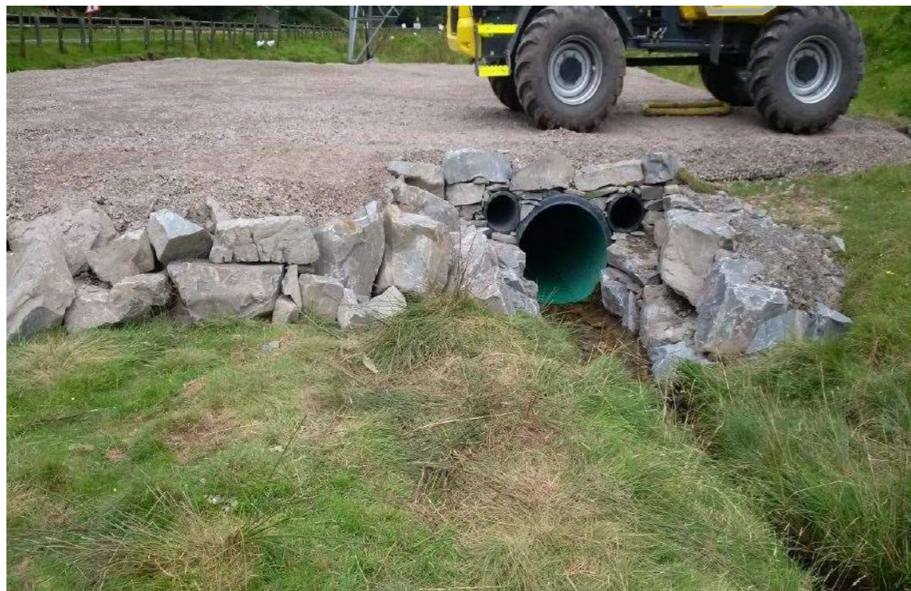
Figure 4.56: Example culvert installed for temporary water course crossing for access
