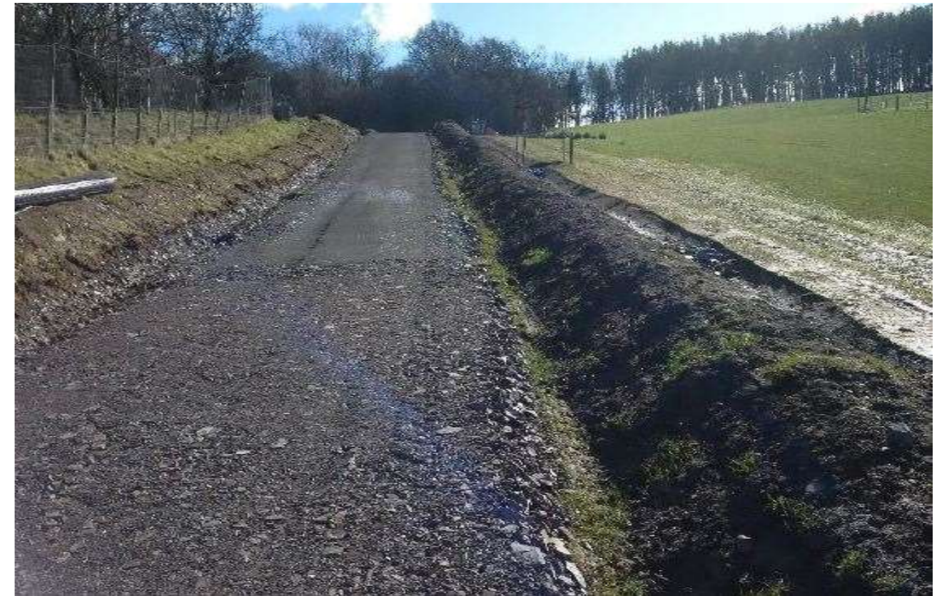
Figure 4.34: Typical stone road installation on top of geomembrane
