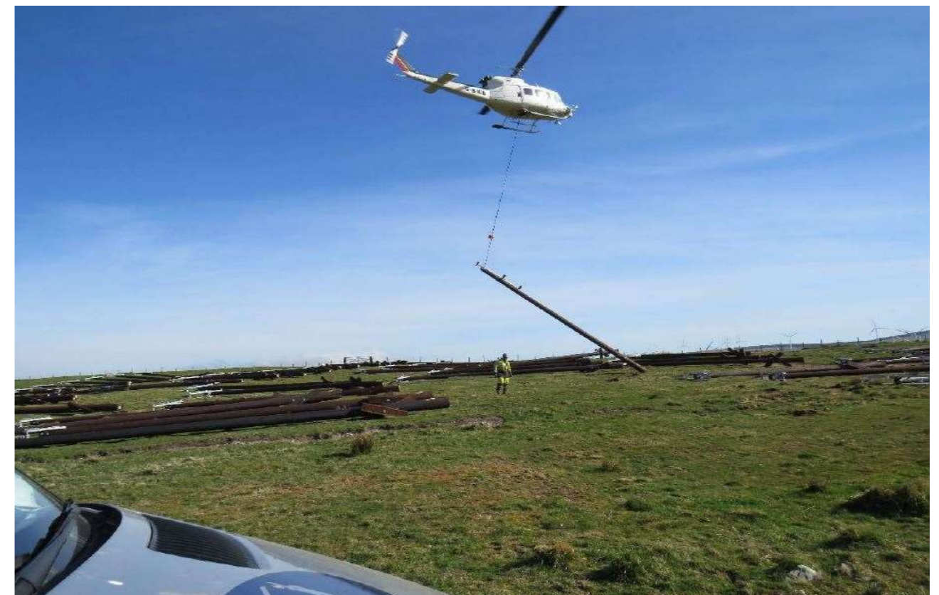
Figure 4.11: Helicopter delivering wood poles to working area
