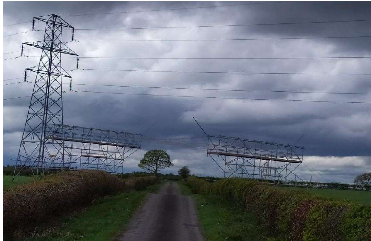
Figure 4.125: Protective scaffolding over road/access track crossing
