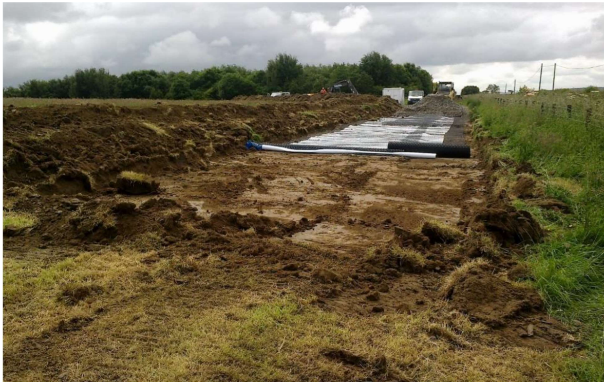
Figure 4.23: Typical stripping and stockpiling of topsoil and laying of geomembrane
