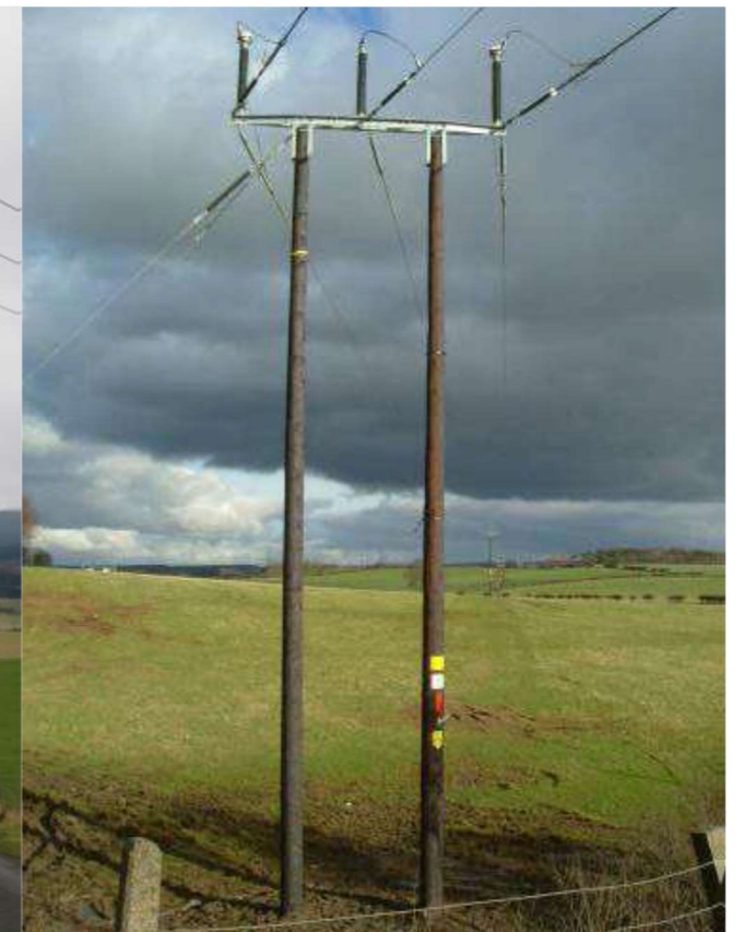
Figure 4.5: Typical angle support-H pole
