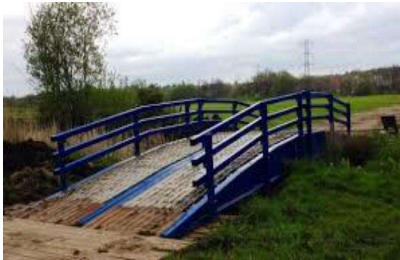
Figure 4.45: Typical temporary bridge for construction vehicle access
