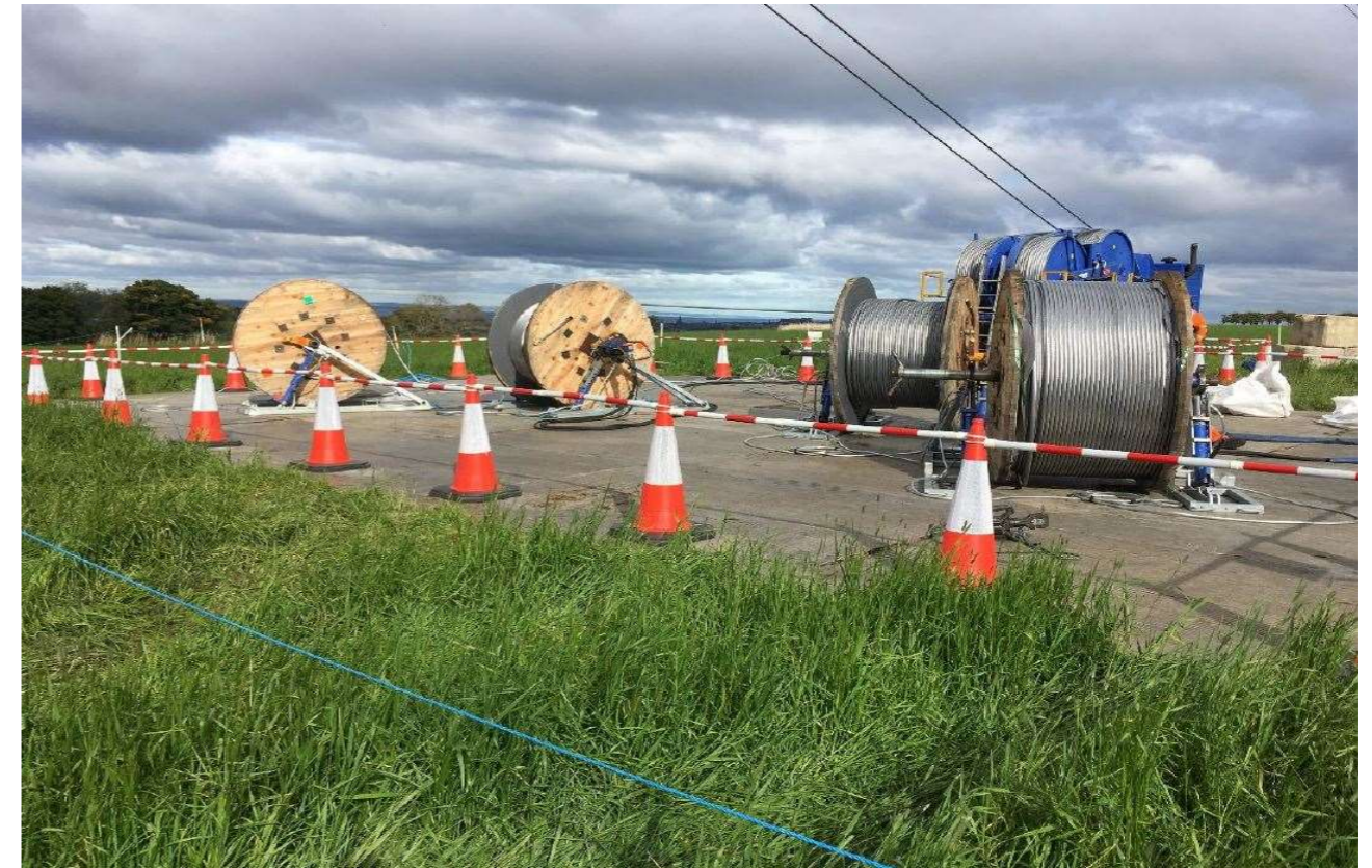
Figure 4.103: Conductor drums and tensioner at tension location
