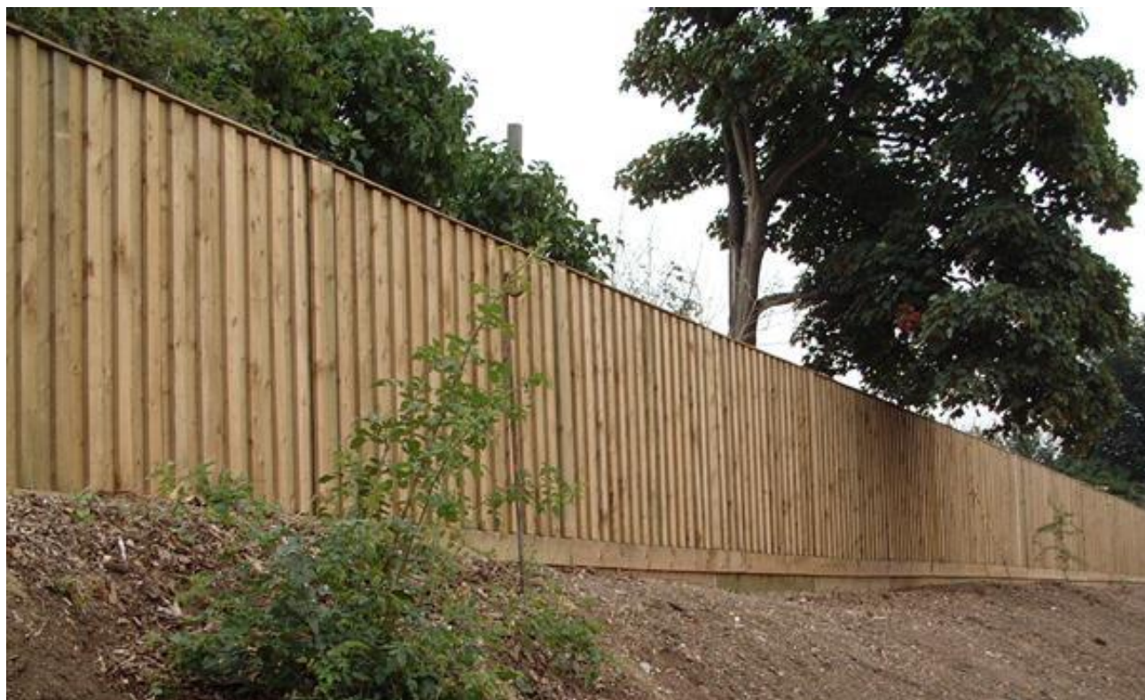
Photo 10.1: Example of a Typical Permanent Noise Barrier 3
