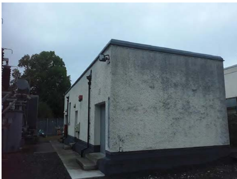
Photograph 1: 'Building 2' with Bat Roost Potential below metal and wooden barge structures
