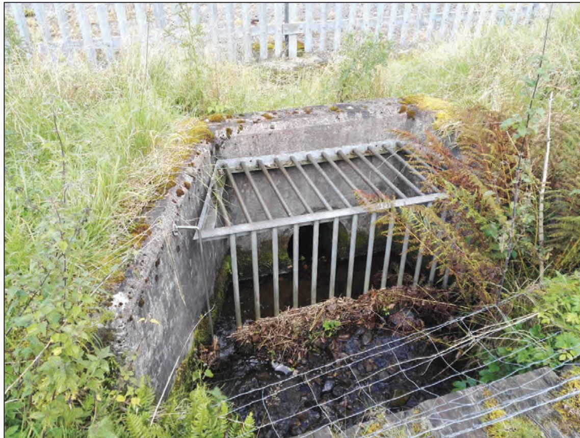
Photo 12: Burn 1 looking downstream at the culvert inlet with wingwalls and trash screen
