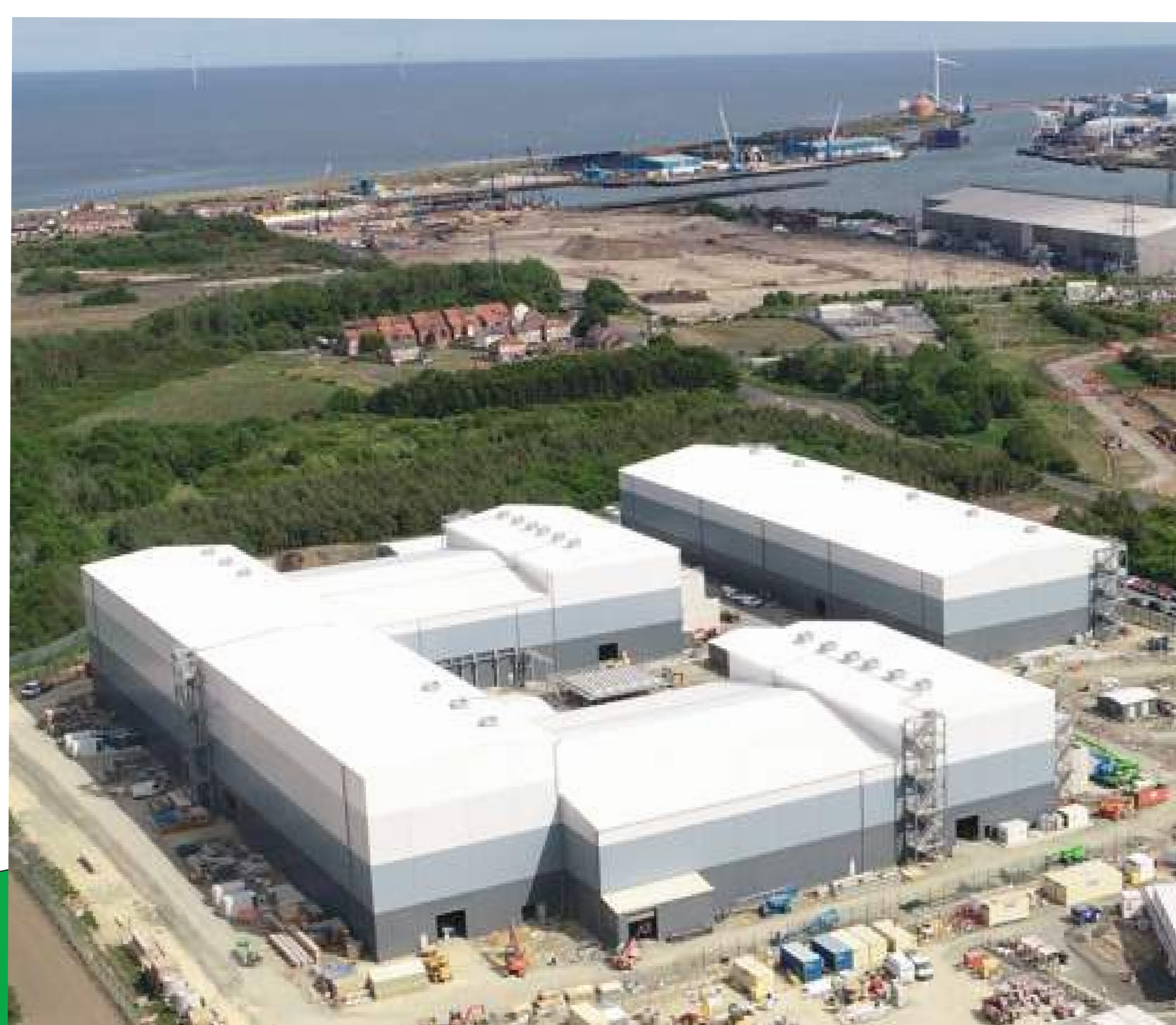
Existing converter station at Blyth, Northumberland
