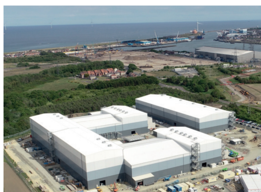
Existing converter station at Blyth, Northumberland
