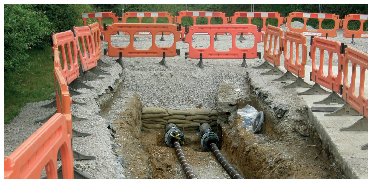
Underground cable installation during construction
