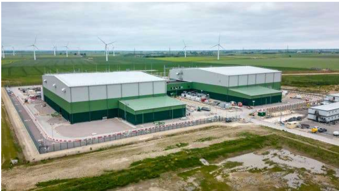
Figure 4 Example of converter station
