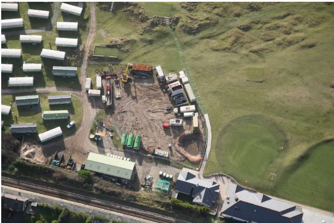
Figure 3 Example of HDD Compound Setup
