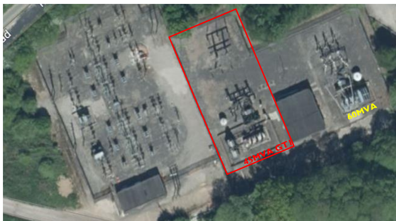
Figure 5.1: Aerial view of Radway Green grid substation
