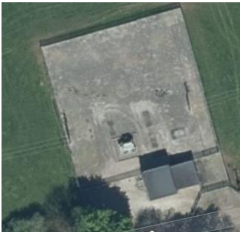
Figure 5.3: Aerial view of existing Weston substation
