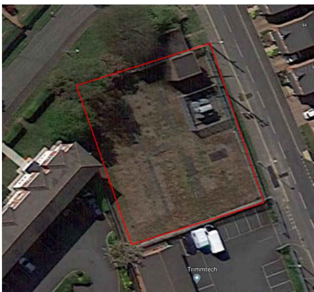
Figure 5. Fodens aerial view
