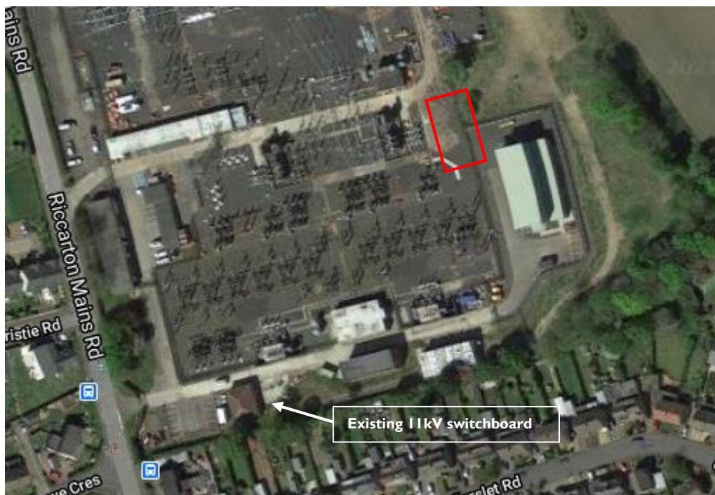
Figure 6. Proposed location for two new 33/11kV transformers at Currie primary
