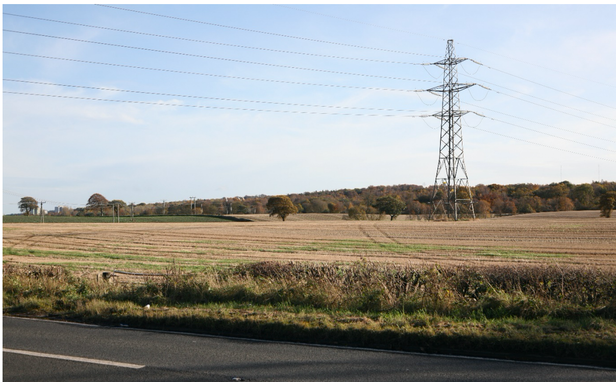
Figure 4 – The double circuit 132kV transmission overhead line between Bonnybridge and Cumbernauld
