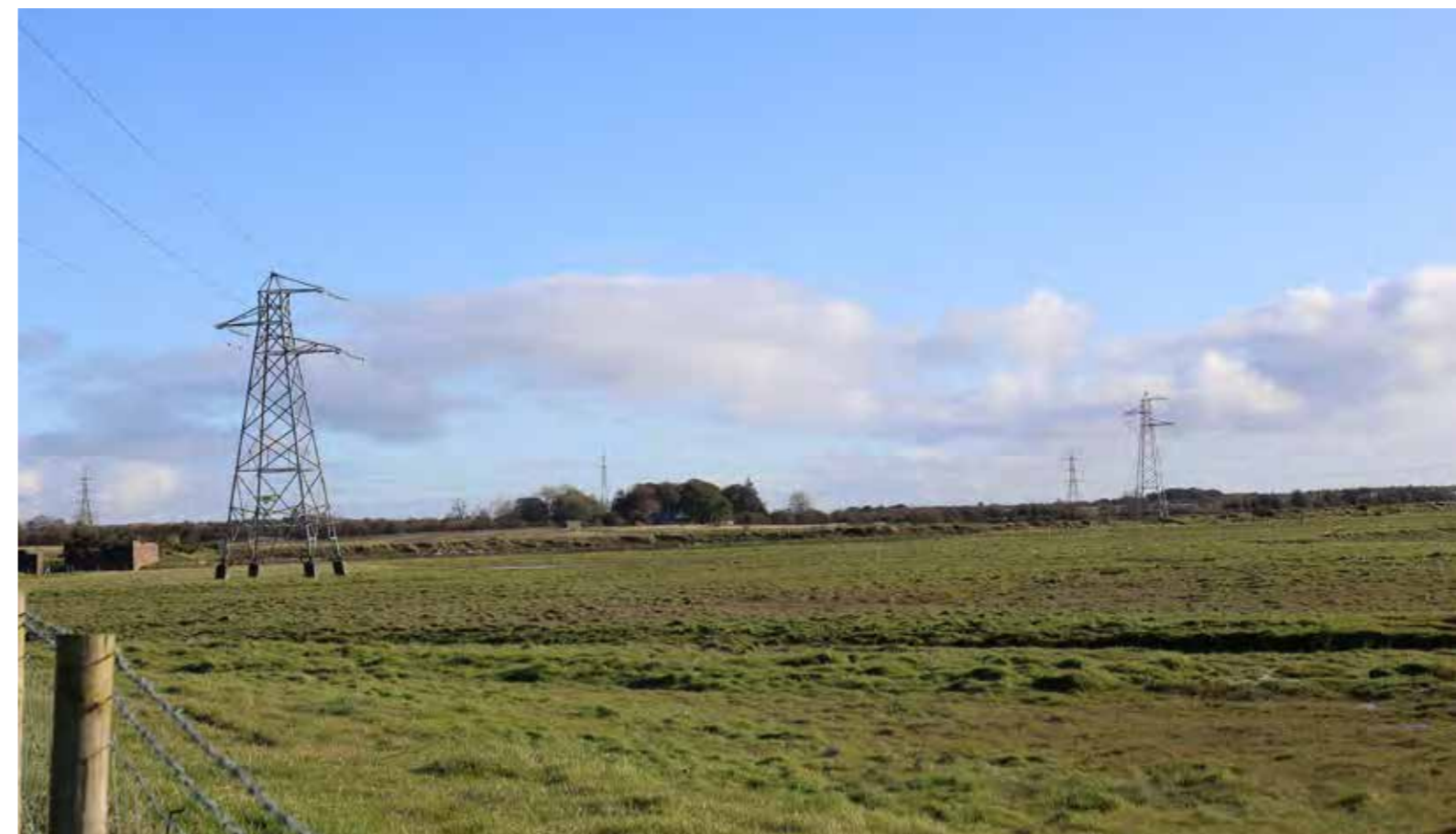
Photo 2: Existing steel towers of T Route
