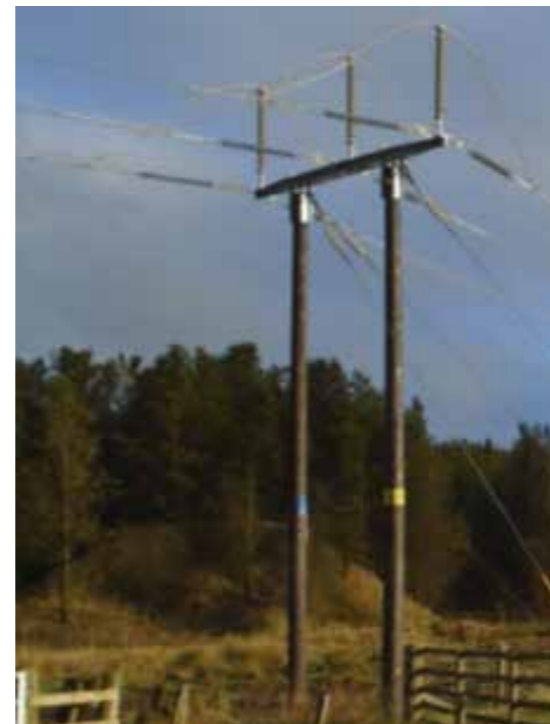
Photo 5: Typical H Pole
