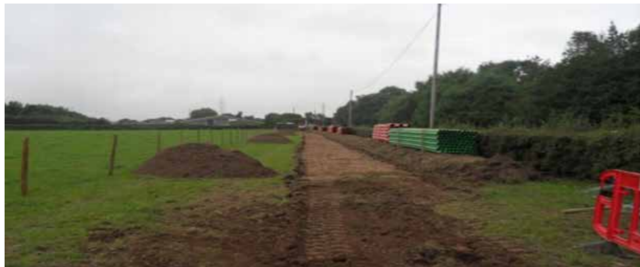
Photo 3: Construction site - laying underground cable
