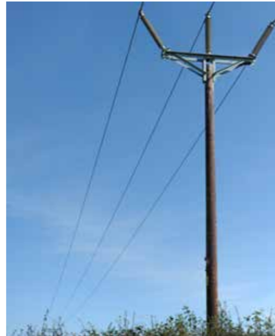
Photo 4: Typical Trident Wood Pole
