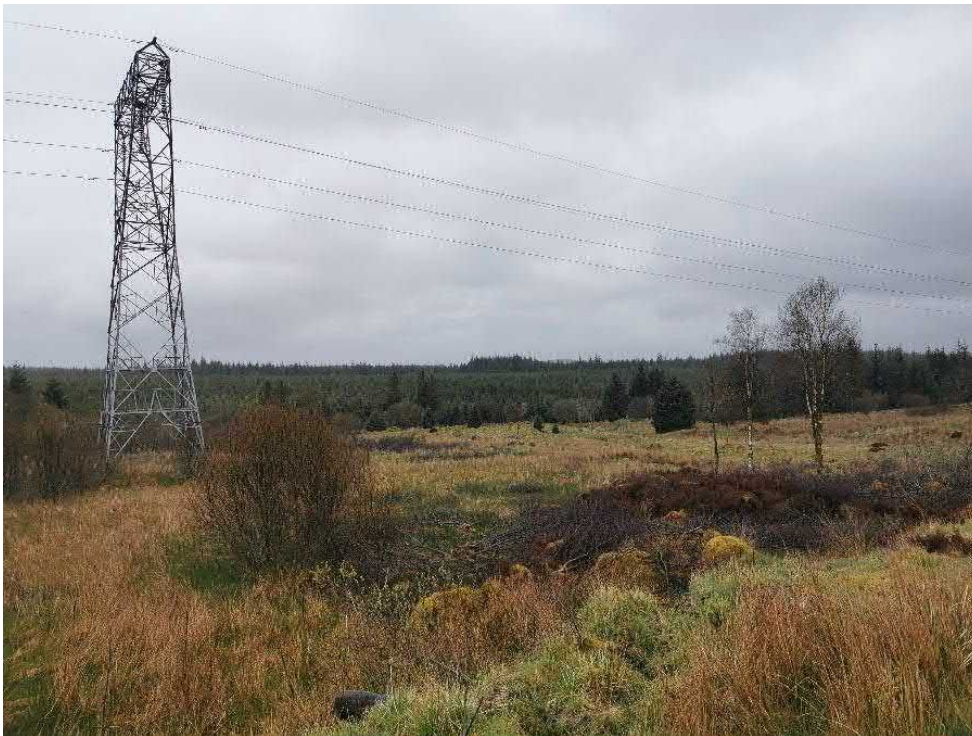
Photo 3-1: Facing towards the proposed location of the Carrick Substation from Carrick Forest Drive
