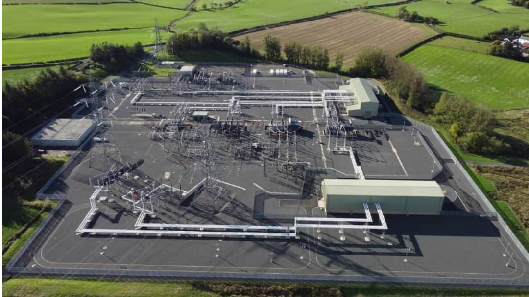
Figure 4 Typical AIS and GIS Substations
