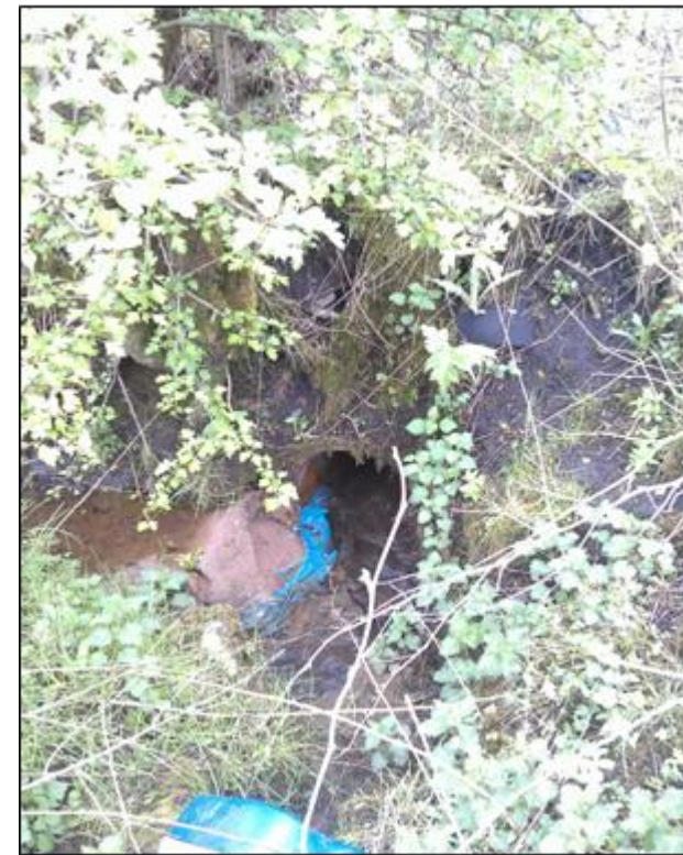
Plate 7.19: Unnamed Watercourse 2 Upstream of the existing culvert crossing
