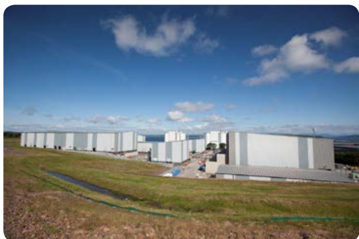
HVDC Converter Station Hunterston
