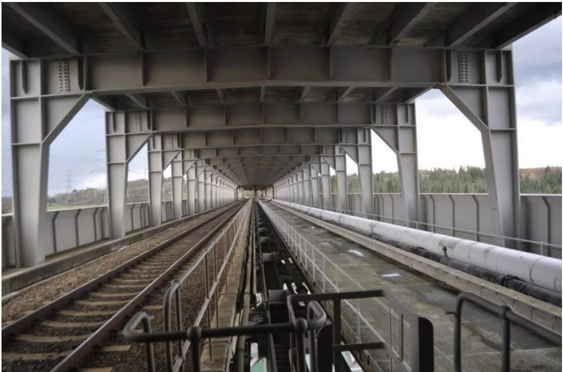
Figure 3-2. Britannia Bridge lower deck showing the proximity of the Bangor to Llanfair AC circuit cables to the railway.
