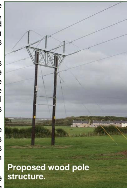
rigidity against the wind speeds to which the structure will be exposed as well as provide greater protection against the potential effects of ice loading. All wood poles are fully seasoned and are treated with an appropriate preservative. At the top of the wood poles the galvanised steelwork structure supports the insulators and three conductors. An earth wire is slung underneath the steelwork.
