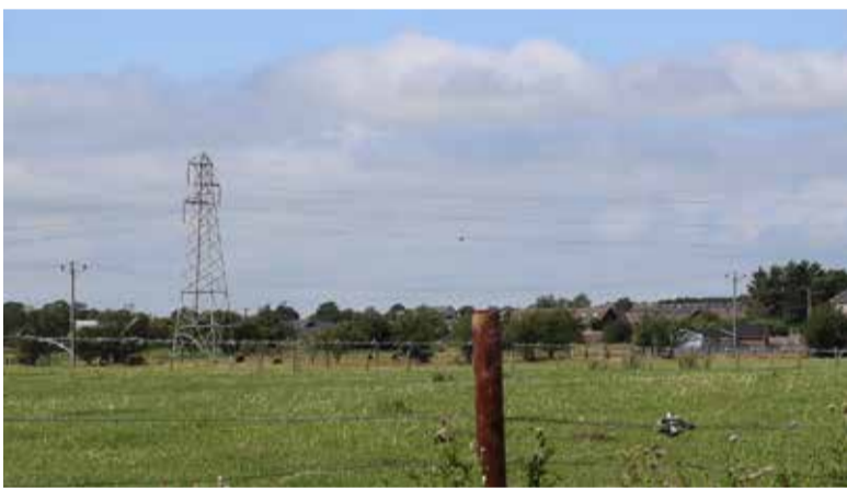
Existing steel lattice tower line forming the T Route
