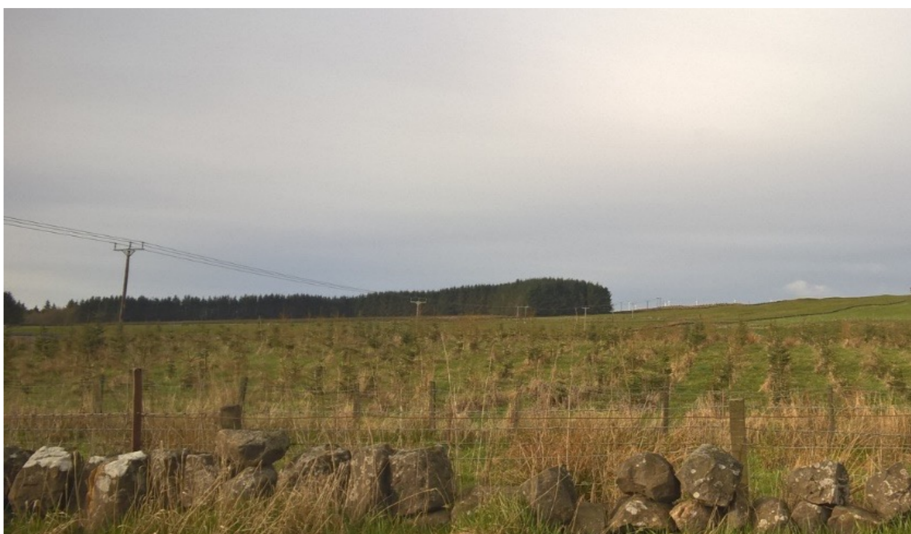
View of existing wood pole OHL south of Coalburn, South Lanarkshire
