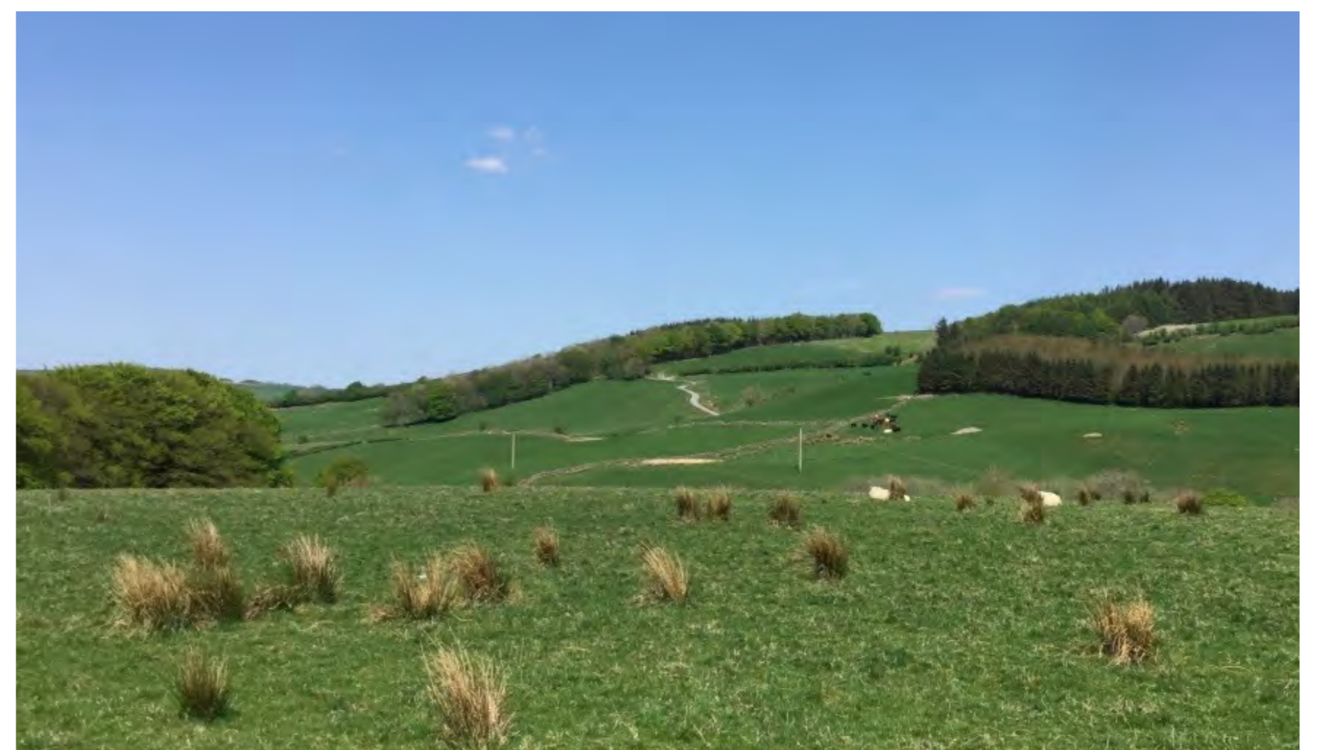
View of existing wood pole OHL in a valley at Chirmorie, south of Barrhill
