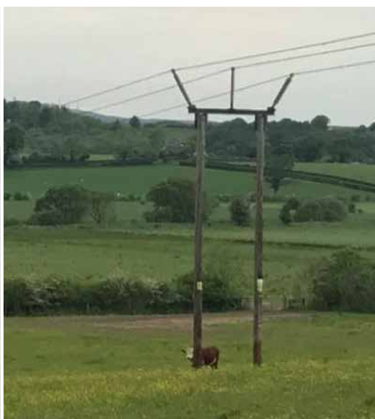
Example of a typical intermediate section of a trident double wood pole supporting a 132-kV OHL (SPEN, 2019)
