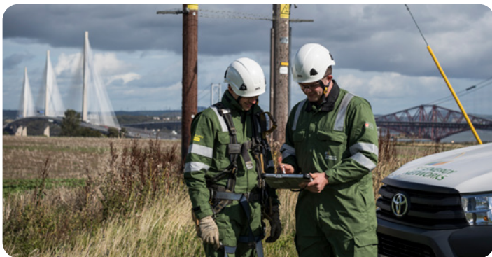
Interruptions incentive example: Maintaining our network and being well prepared for severe weather events.
